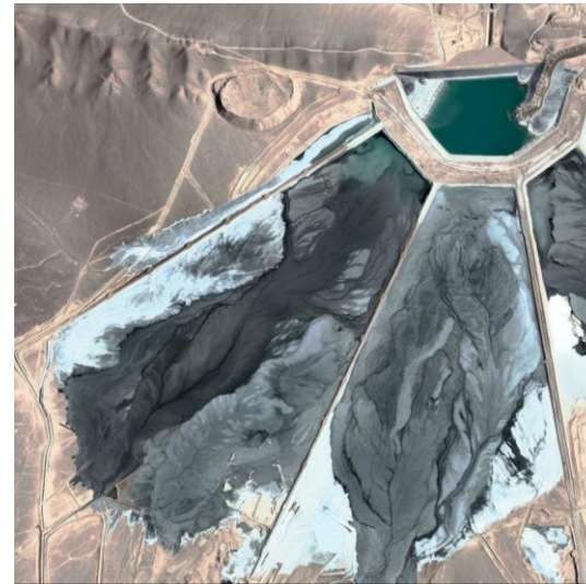
Tailings Storage Facility
